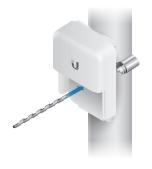
2. Drill a pilot hole into the pole.
