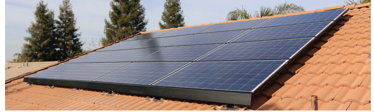
Four Landscape Trim Covers Installed
